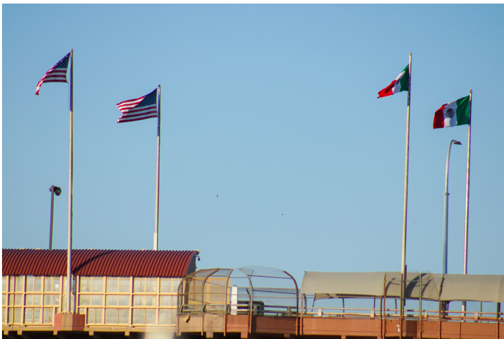
The Córdoba Bridge of the Americas between Juárez and El Paso.
